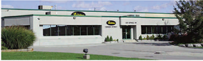
Fairview Fittings & Manufacturing Limited Canadian Head Office / Distribution Centre Toronto Canada
